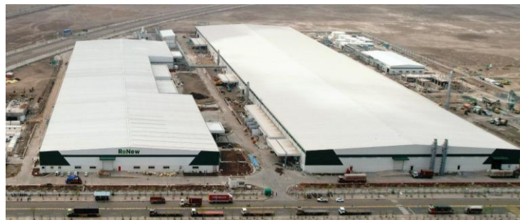
Dholera module plant (2.4 GW)
