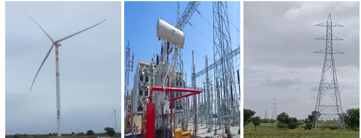
Round the Clock (RTC) Power Project
