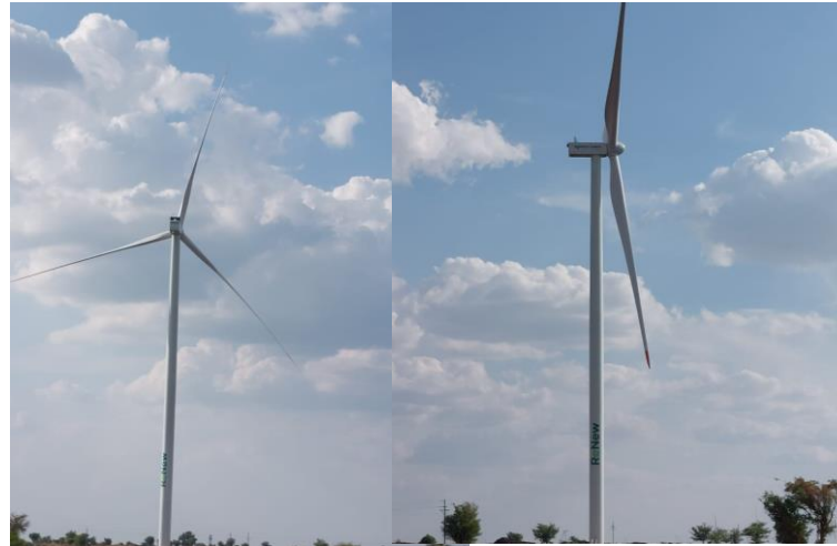
Round the Clock (RTC) Power Project
